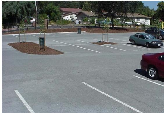
*Pervious pavements function like storm water retention basins and allow the stormwater to infiltrate the soil over a large area, thus facilitating recharge of precious groundwater supplies.*
